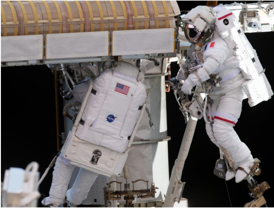
Spacewalkers Shane Kimbrough, left, and Thomas Pesquet work to complete the installation of a roll-out solar array on the International Space Station. Picture: NASA.
